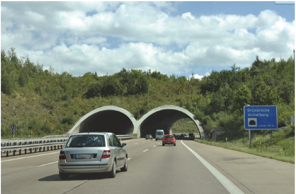
Figure 2.5: Wildlife Bridge over a federal motorway in Germany (Photo: Sarah. Walz)
