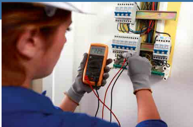
1 Electrician carrying out measurements with a multimeter
