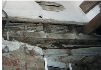
Figure 5.18: Timber beam with 12x 16 cm dimensions is placed above the steel beam. A masonry wall of the basement floor and bagdadi laths from a wall of the ground floor are also seen.
