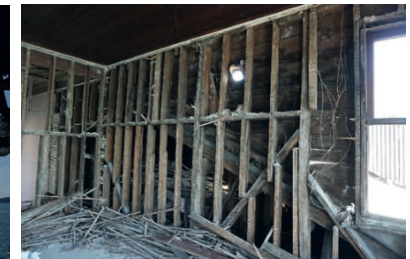
Figure 5.41: Scene from the hall of the top floor showing the ceiling and structural system of the walls.
