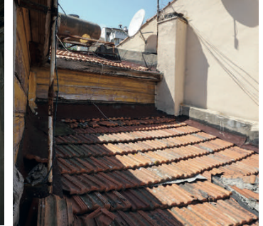
Figure 5.16: Leveled roof and the tiles
