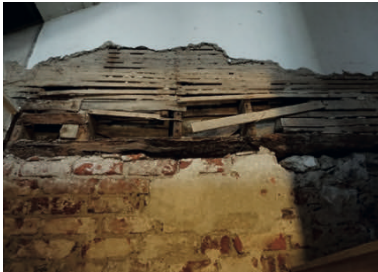
Figure 5.19: Timber beam above the masonry basement. Studs are 4x 13 cm and damaged beam is approximately 12x13 cm. Timber bagdadi laths and plaster are also visible.
