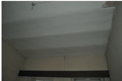
Figure 5.44: Jack arch system
