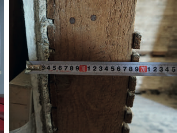
Figure 5.39: Wall thickness and the layers of the wall
