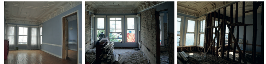
Figure 5.52: Different layers of the same wall in the hall of the second floor. The photos were taken between 2015-2017 by the author before and during the restoration work.
