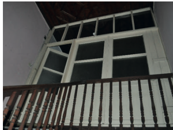
Figure 5.33: Dividing panel as a later application
