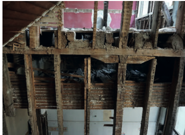
Figure 5.46: Structural system and another cushion beam
