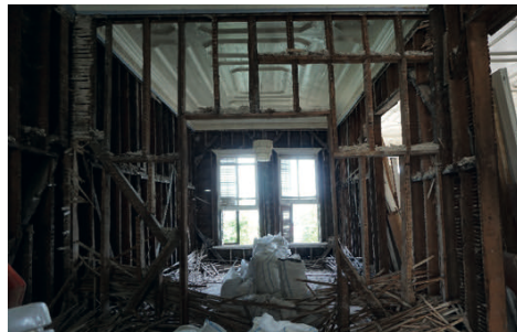
Figure 5.48: Constructive wooden elements of the walls
