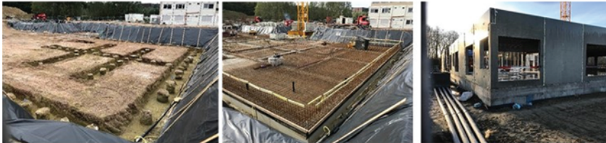
The contractor builds
