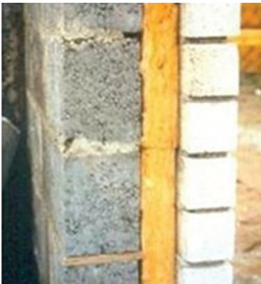
Figure 1.7 Filled cavity wall.
