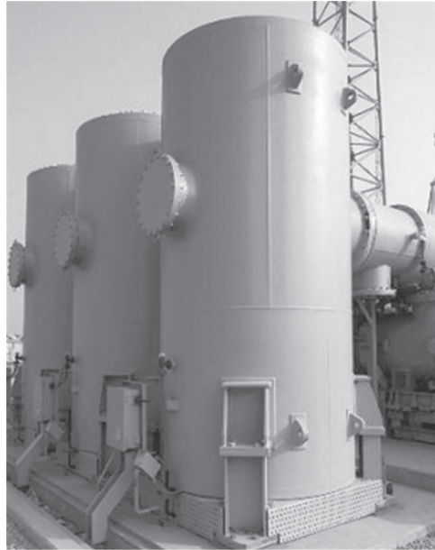
Figure 1.11 Ultrahigh voltage AC tank-type surge arresters in 1000 kV Jindongnan Substation in China.
