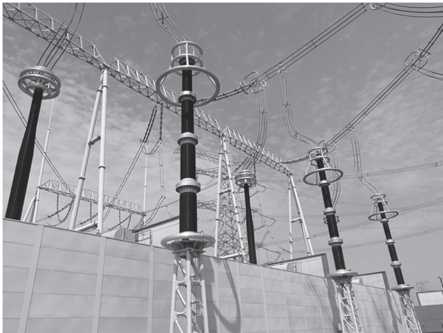
Figure 1.9 1000 kV ultrahigh voltage AC surge arresters with porcelain houses in Dongwu 1000 kV UHV AC substation. Source: Courtesy of X. Zhao.
